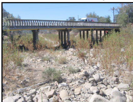
View downstream at the Grand Ave. bridge
