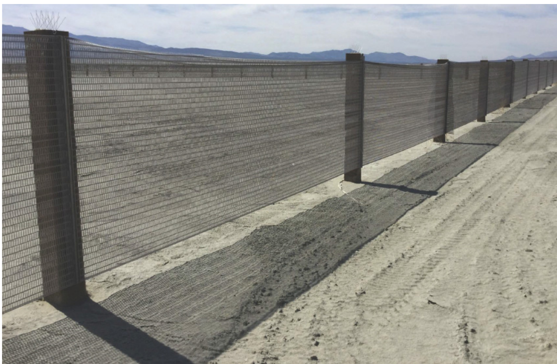
FIGURE 6-5 Sand fence at Owens Lake. SOURCE: LADWP. Photograph by Mark Schaaf, Air Sciences.
