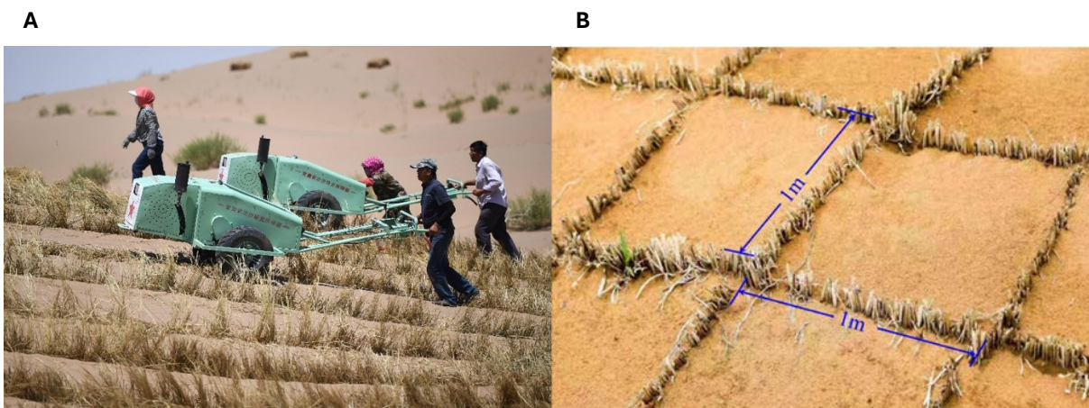
FIGURE 6-3 A) Gasoline powered machines insert straw to form straw checkerboard barriers. B) Sand dunes in western China covered by straw checkerboard.
