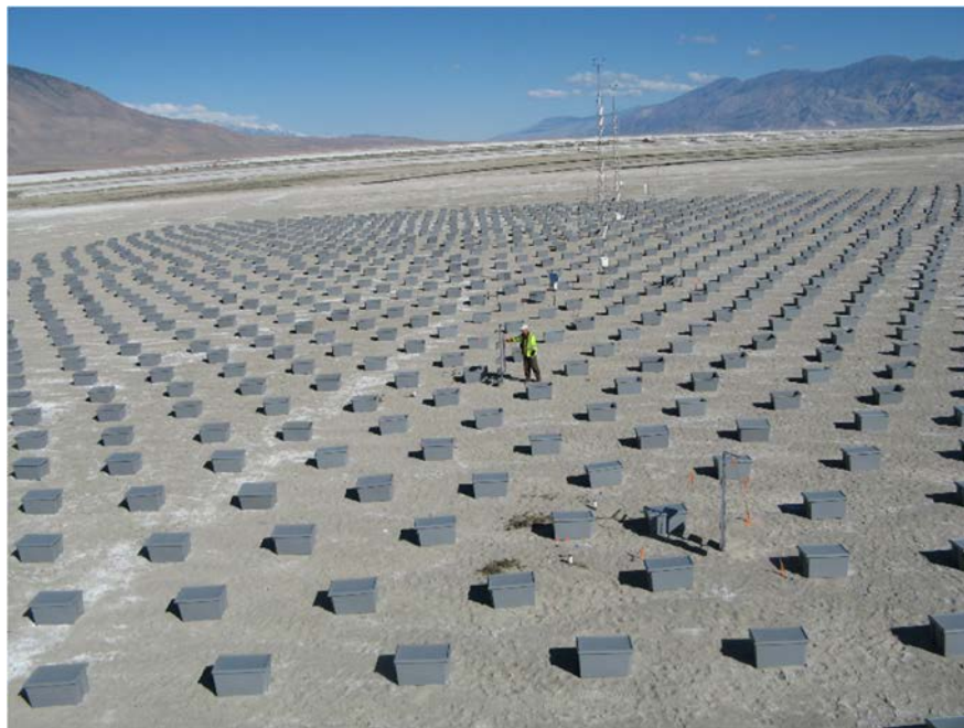
FIGURE 6-4 Weighted plastic totes used as engineered solid roughness objects on Owens Lake. SOURCE: Grace Holder, GBUAPCD, personal communication, August 2019.
