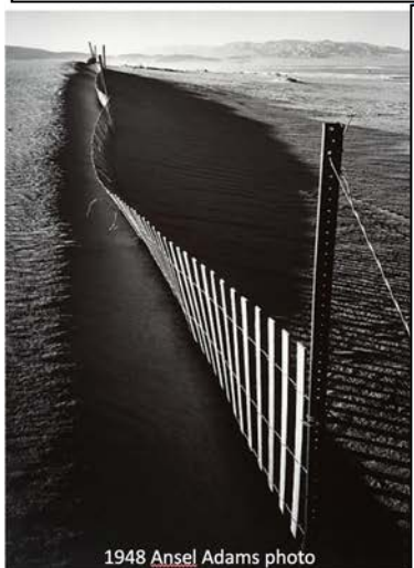
FIGURE 4-11 Historical photos after lake desiccation but before construction of highway berms, showing active dunes associated with significant aeolian transport necessitating installation of sand fences to protect Highway 136 before it was relocated further up Keeler/Slate Canyon fan. SOURCES: Upper location map by G. Holder, GBUAPCD, personal communication, May 29, 2024; 1934 and 1949 photos from CalTrans; 1948 photo by Ansel Adams; 1953 courtesy of Dennis Burke.
