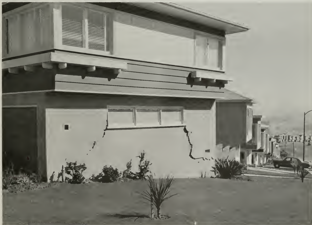
Photo 2. House damaged by earthquake of March 22, 1957, Westlake Palisades area, Daly City.
