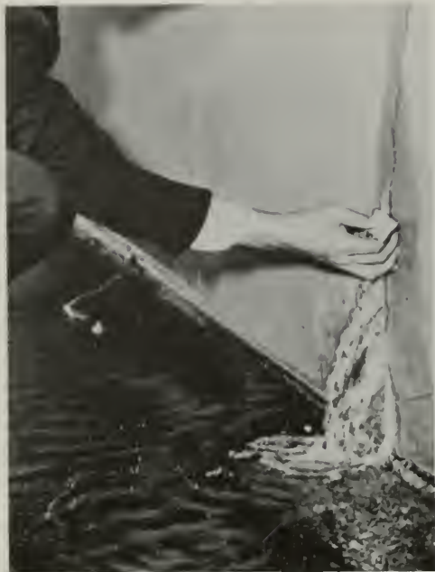
Photo 2. Leak in east wall of Westlake Palisades Reservoir developed during 1957 earthquake. Photograph courtesy of San Francisco Examiner.
