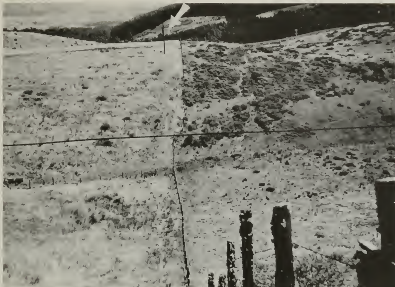
Photo 4. Fence that was ruptured, bent, and shifted badly more than 5 feet by movement of the San Andreas fault in 1906. Solid line shows trace of fault. Arrow points to building that is also shown in photo 5. Photograph taken in 1956.
