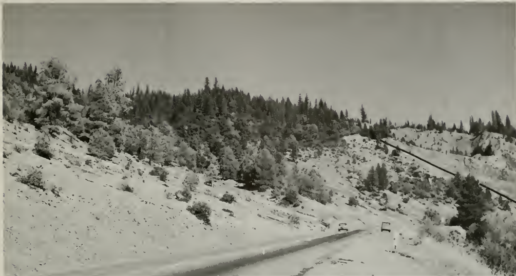
Photo 6. View of La Grange fault, looking northeast along U. S. Highway 299 in northwest corner of Weaverville quadrangle. Hillside to left of highway is exhumed footwall surface of fault, consisting of Salmon Schist with thin capping of mylonite. Approximate dip-slope trace of fault is shown by black line in right background. Rocks in background beyond trace of fault are chiefly highly-sheared Abrams Schist of hanging-wall block.
