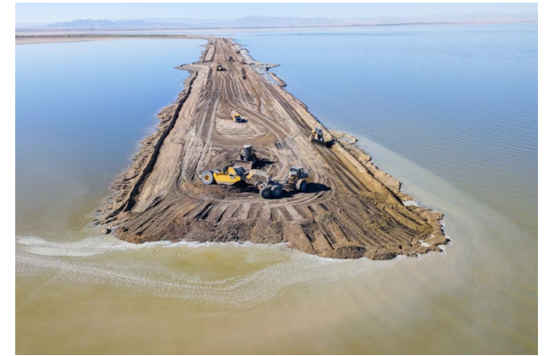
Figure 6. Construction of the SCH Expansion East Pond 1 berm.
