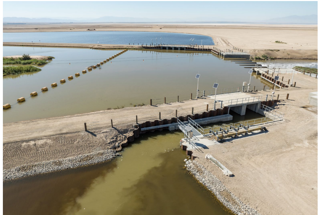
The New River diversion structure at the SCH Project.
