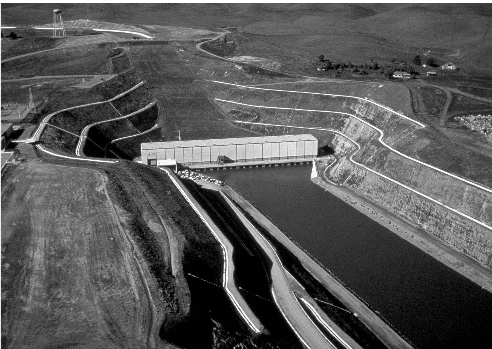
Banks Pumping Plant
