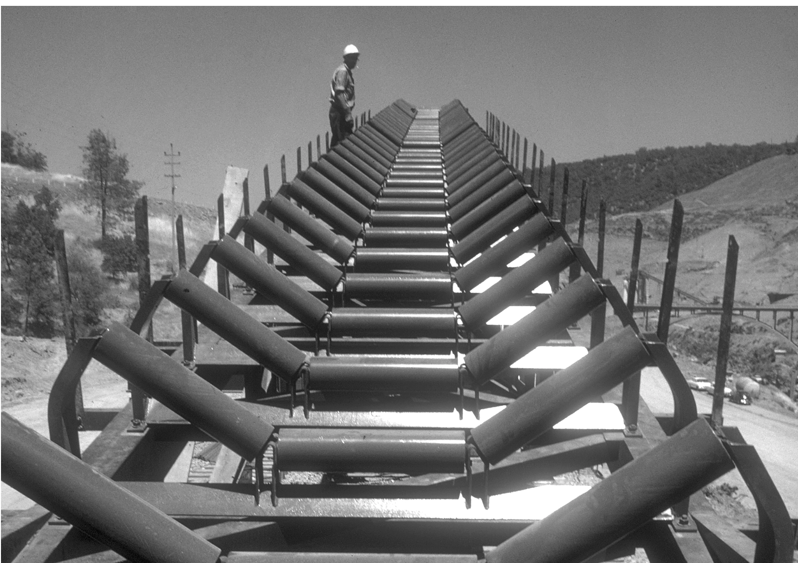
Construction at Oroville Dam
