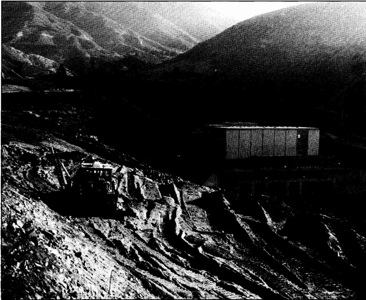
The enlargement of Devil Canyon Powerplant is scheduled to be completed in 1992.
