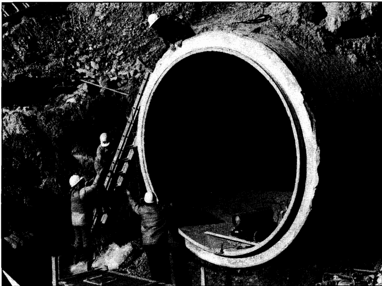
The Mojave Siphon Pipeline, which ruptured on November 9, 1988, was returned to service on November 25, 1988 after repairs had been completed.
