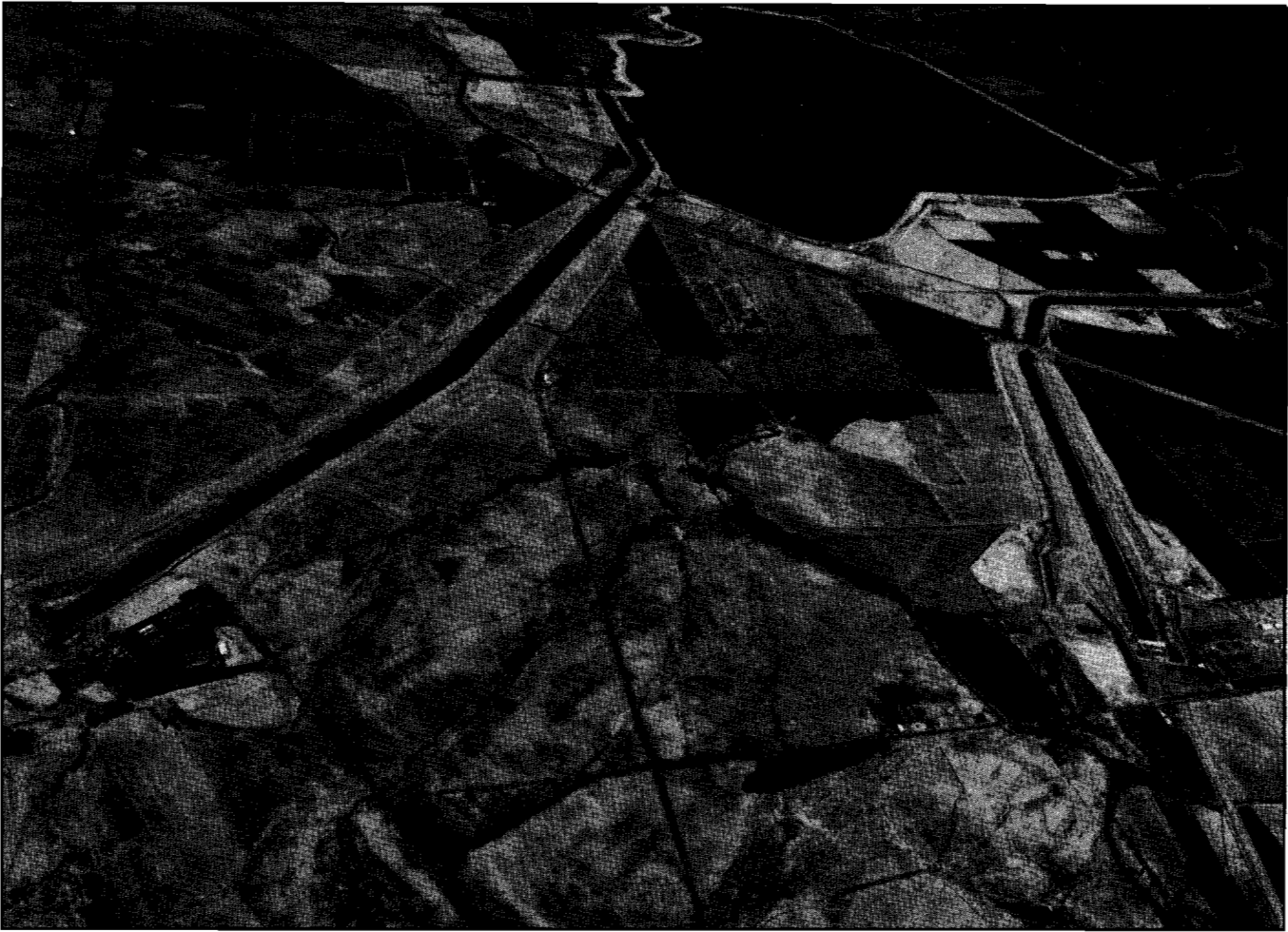
Under the COA, DWR pumped 193,590 acre-feet of CVP water at Banks Pumping Plant (left) during 1988 to replace USBR capacity foregone at Tracy Pumping Plant (right).
