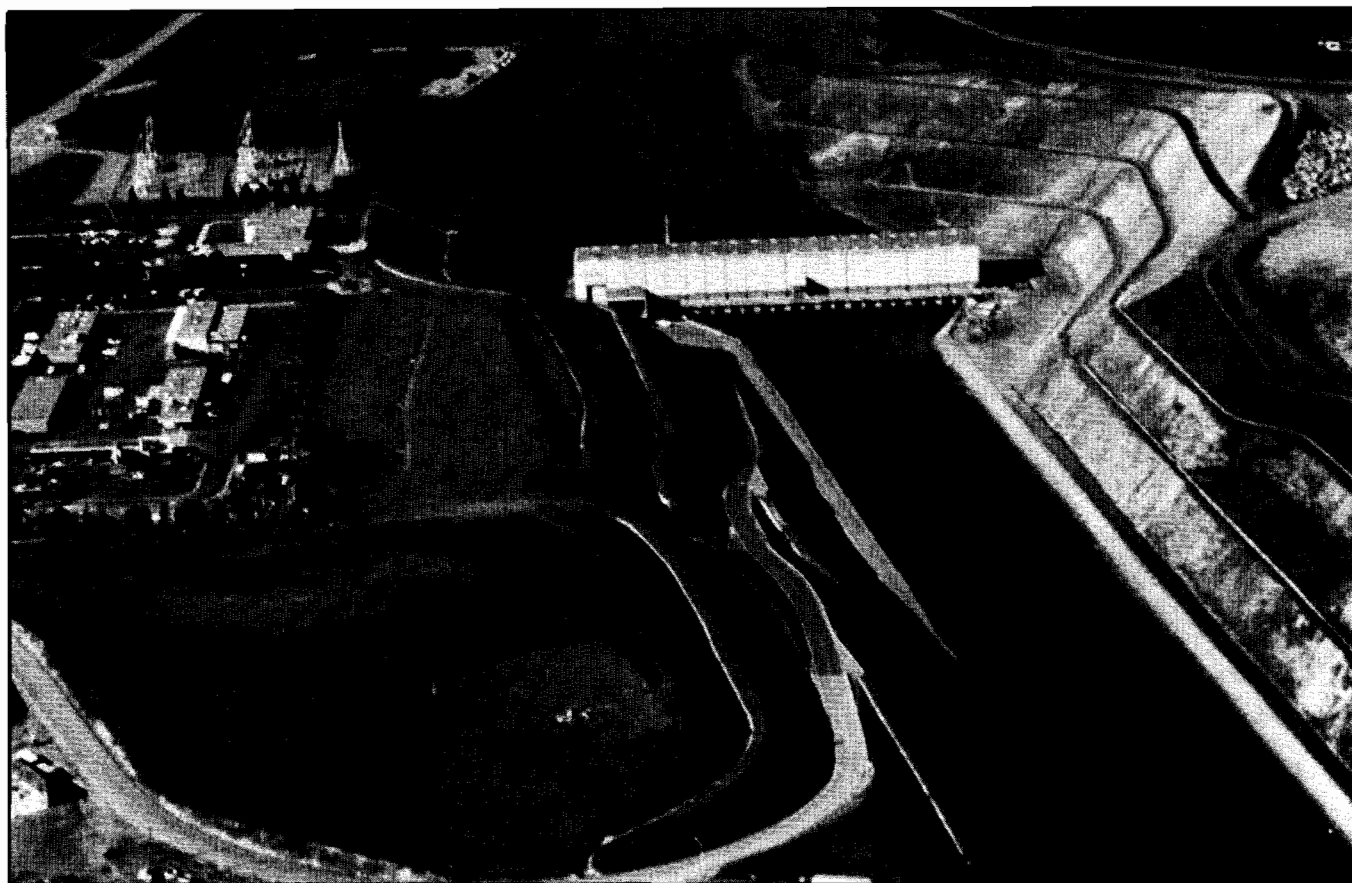
Construction continues for the enlargement of Harvey O. Banks Delta Pumping Plant.
