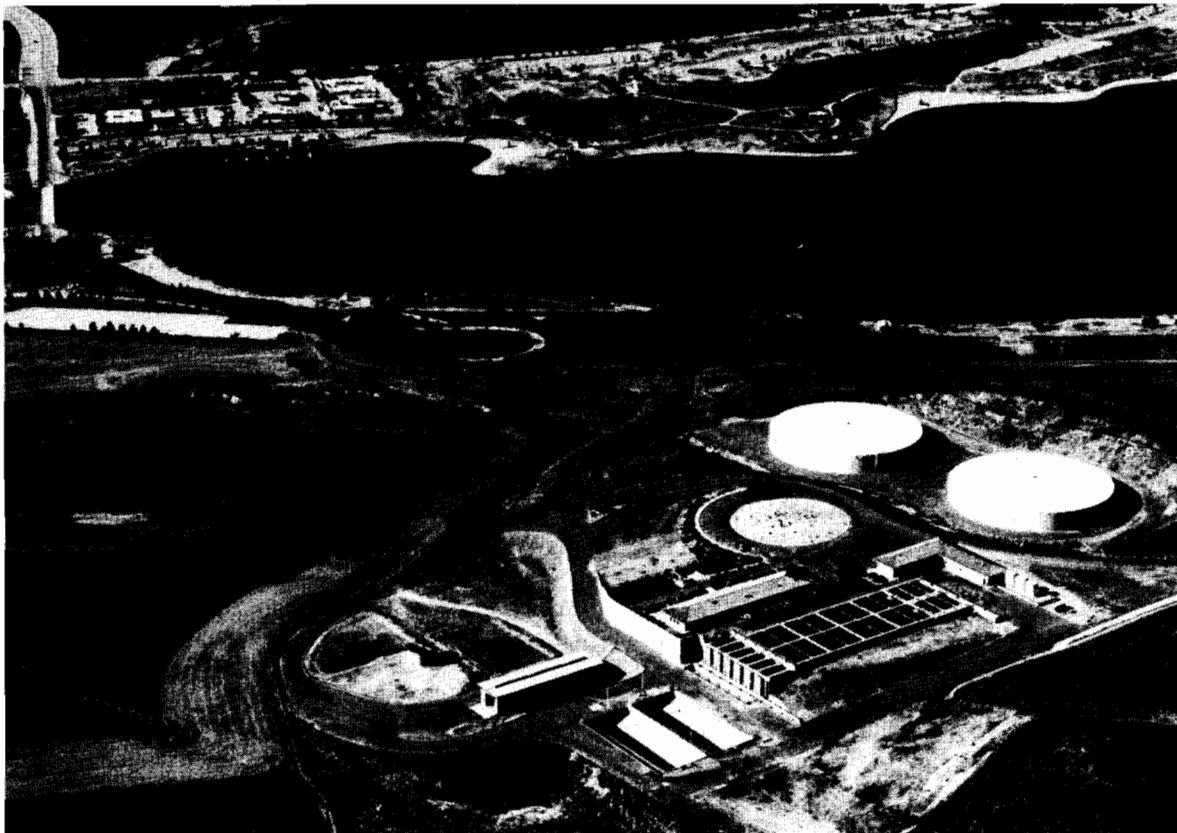
CLWA's Earl Schmidt Filtration Plant, near Castaic Lagoon, can treat up to 12.5 million gallons per day; the installation includes two 5-million gallon storage tanks.
