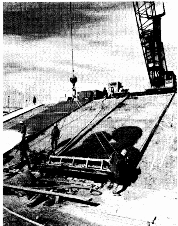
Lining the transition channel downstream of Alamo Powerplant
