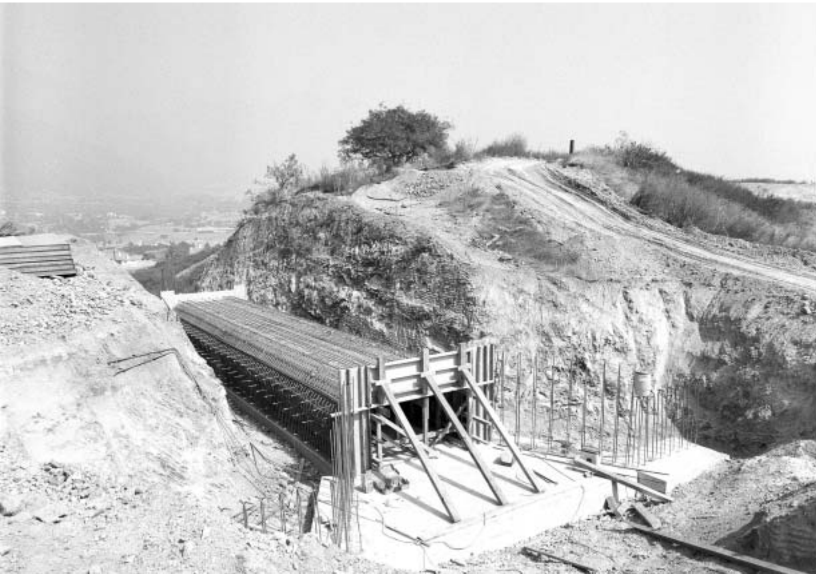
Spillway structure for Crafton Hills Reservoir of the East Branch Extension
