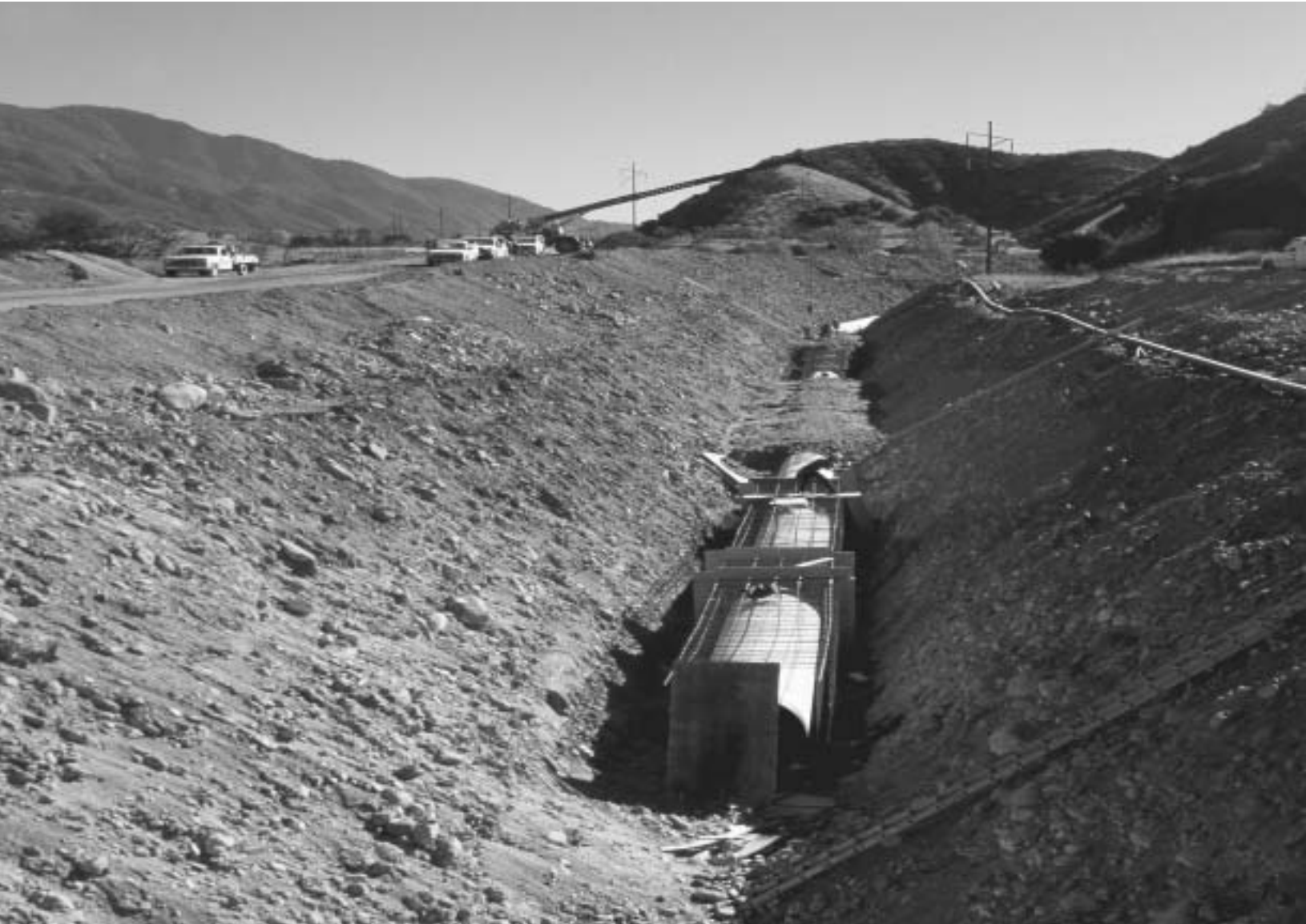
Segment of the East Branch Extension Phase I, Reach 1, winding its way to the Crafton Hills Reservoir
