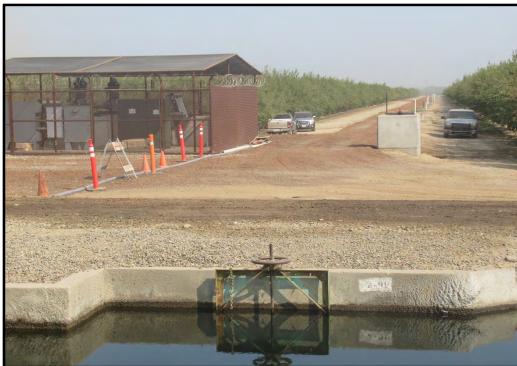
Outlet from the MID lateral and adjacent groundwater well that provide water to Riley Slough via a pipeline, looking north; 09/15/21.
