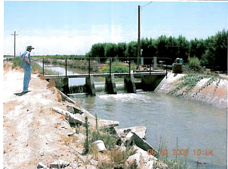
Drop structure in Banks Ditch.
