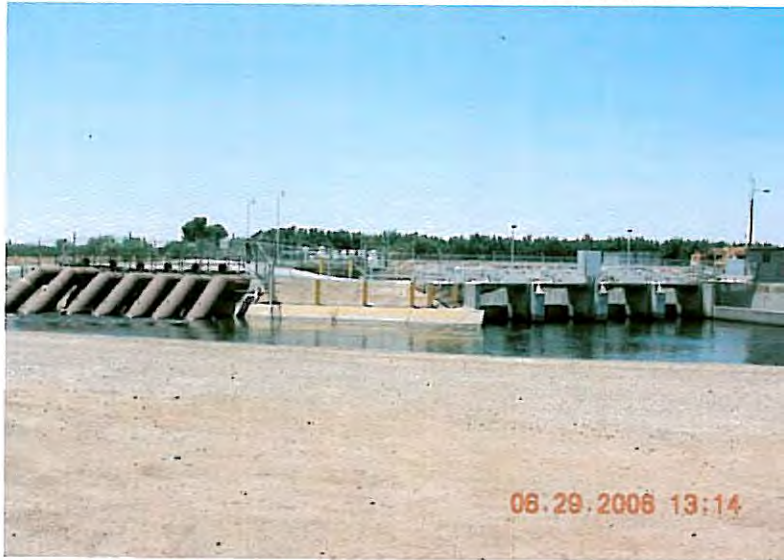
Permanent pumps in the Tule River Wasteway used to move water from the Tule River into the Friant-Kern Canal.
