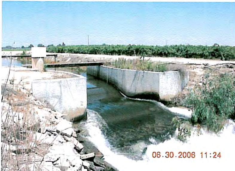
Flume on unnamed canal near People's Ditch.
