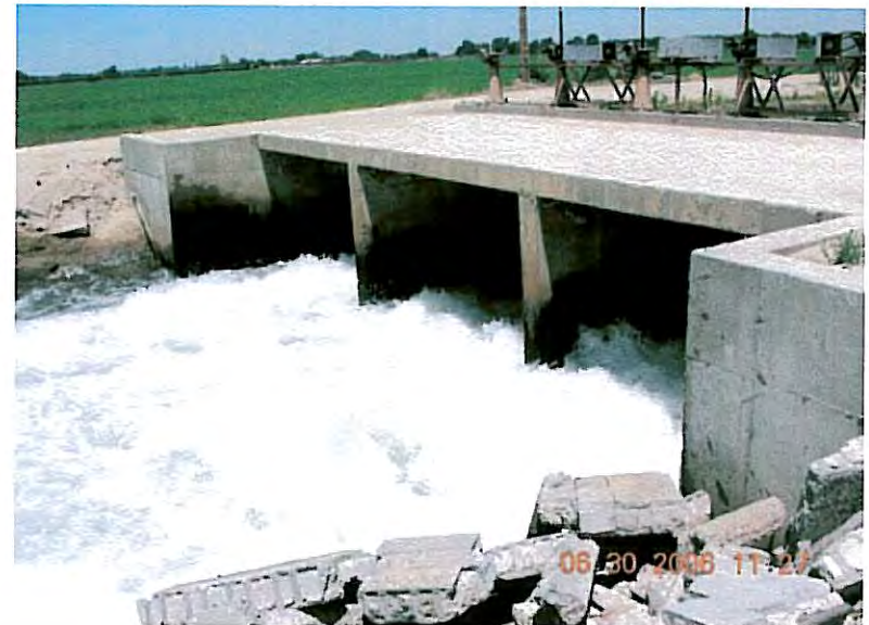
Drop structure in People's Ditch.
