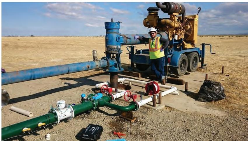
**Figure ES-3. Wellhead Control and Other Equipment**
