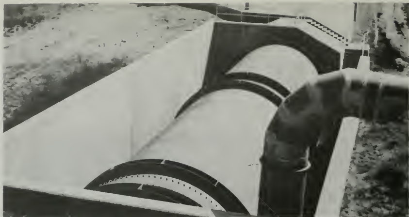
Figure 358. Outlet Works Turnouts
