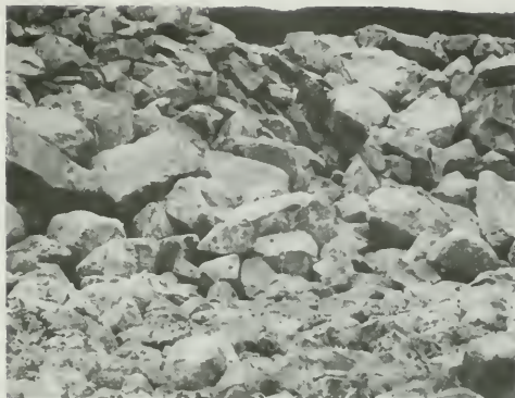
Figure 275. Zone 5 Embankment Shell Material
