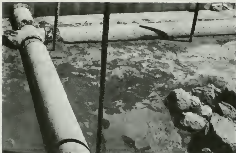
Figure 263. Perforated Drain Pipes in Spillway Chute
