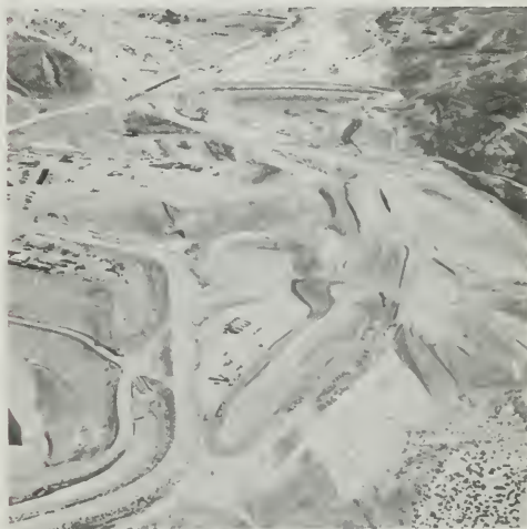
Figure 383. Dam Site at Beginning of Work
