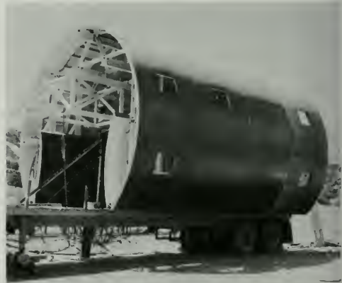
Figure 225. Tunnel Crown Placement Forms
