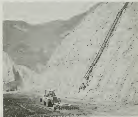
Figure 325. Presplit Face of Shaping Area on Right Abutment
