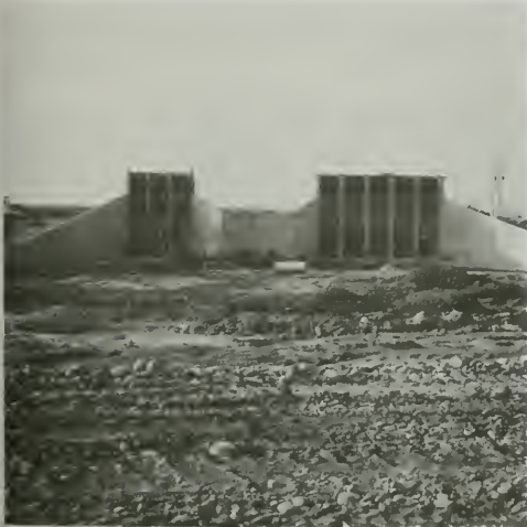
Figure 165. Western Canal and Richvale Canal Outlets—Upstream View
