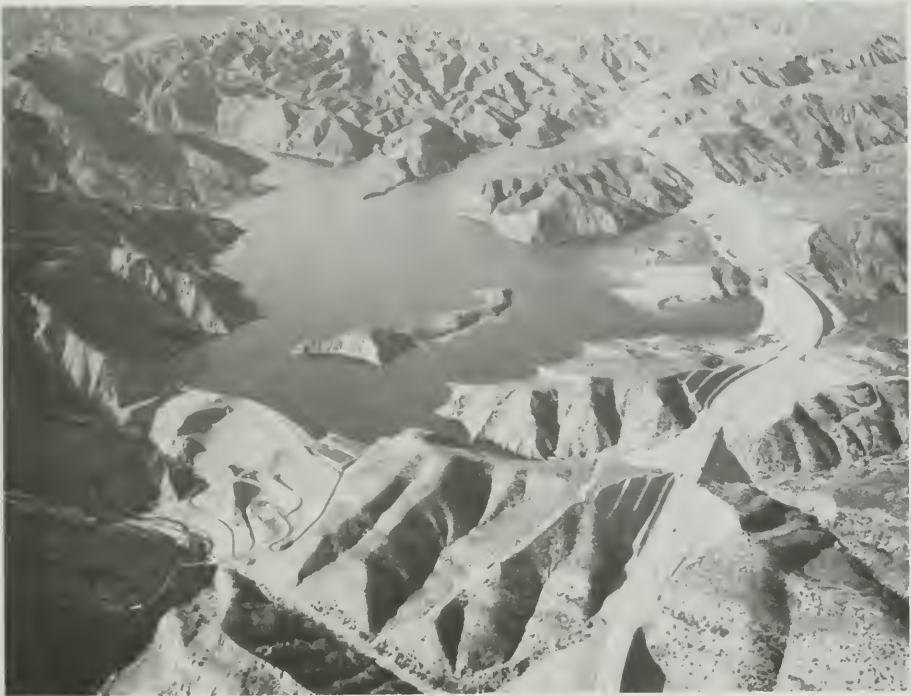
Figure 301. Aerial View—Pyramid Dam and Lake
