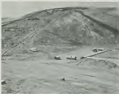
Figure 199. Foundation Grouting—Bethany Forebay Dam
