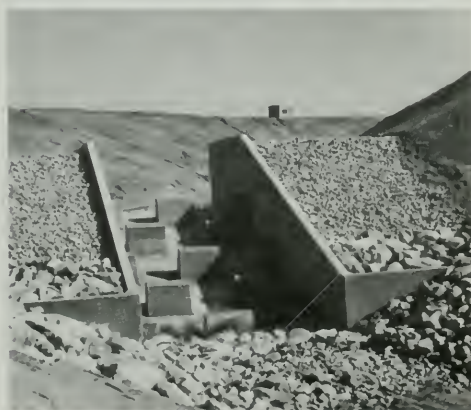
Figure 299. Concrete Placement in Spillway
