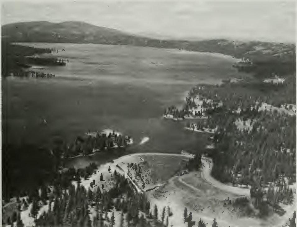
Figure 41. Aerial View—Grizzly Valley Dam and Lake Davis
