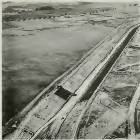
Figure 163. Bedding Placement on Tail Channel
