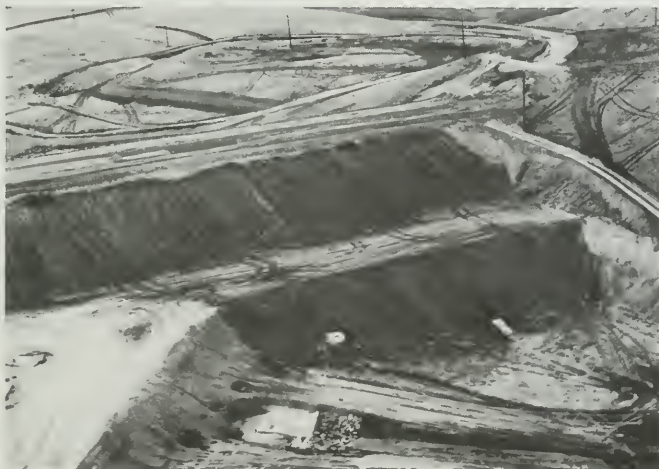
Figure 201. Bethony Forebay Dam Construction
