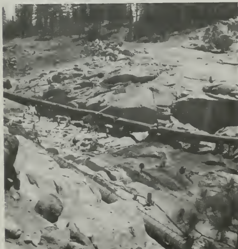
Figure 34. Temporary Diversion Pipe and Outlet Works Conduit
