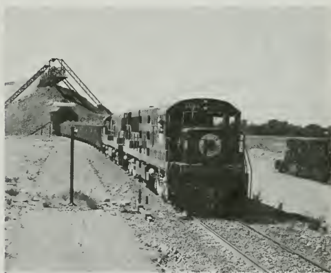
Figure 105. Pervious Loading Station
