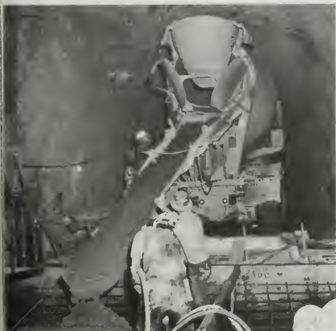
Figure 277. Placing Concrete in Gate Chamber
