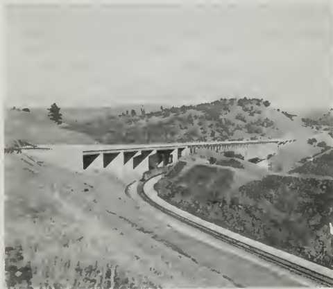
Figure 89. West Branch Bridge
