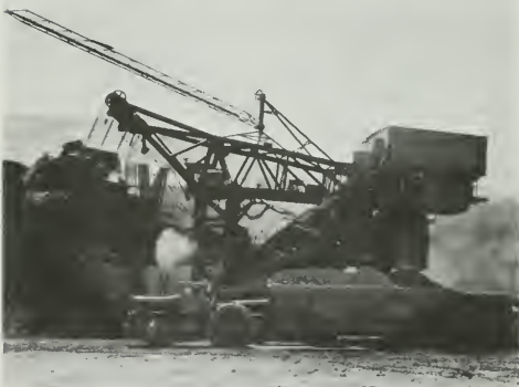
Figure 234. Wheel Excavator Cutting on 50-Foot-High Face
