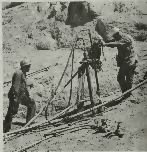
Figure 35. Drilling Grout Hole—Left Abutment Auxiliary Dam
