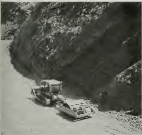
Figure 331. Compacting PerVIOUS Material With 10-Ton Vibratory Roller
