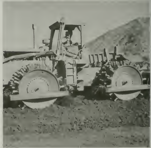
Figure 330. Rolling of Impervious Fill
