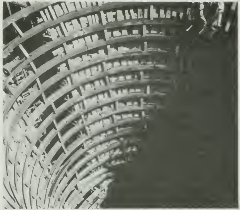
Figure 224. Spillway Shaft Excavation Support
