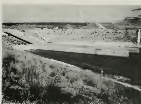
Figure 343. Outlet Works Energy Dissipator
