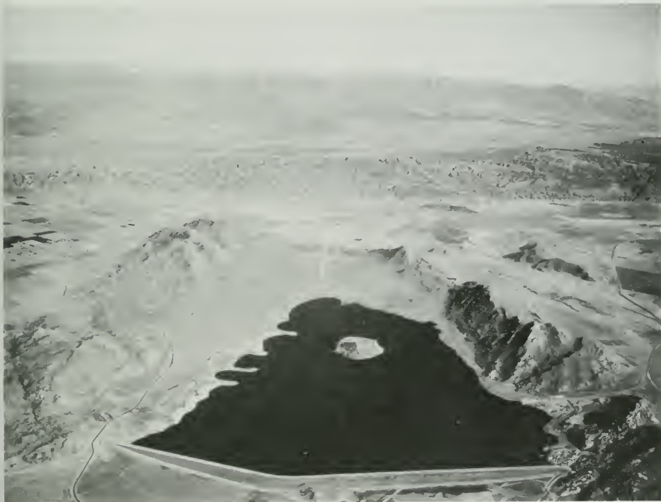
Figure 279. Aerial View—Perris Dam and Lake Perris
