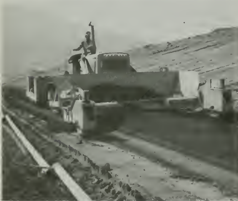
Figure 391. Spreading Soil-Cement
