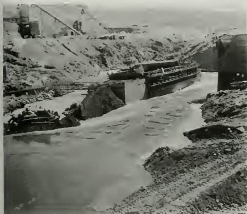
Figure 95. Stage 2 Diversion Earth Dike
