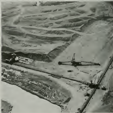
Figure 103. Initial Set-Up of Excavation
