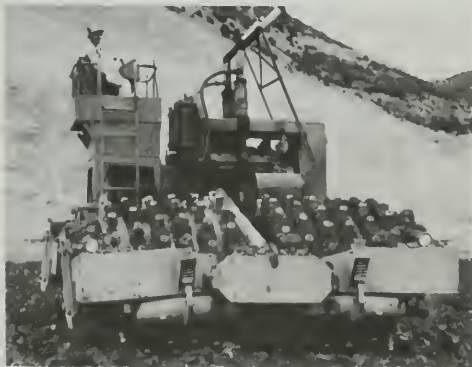
Figure 272. Compacting Zone 1 Material
