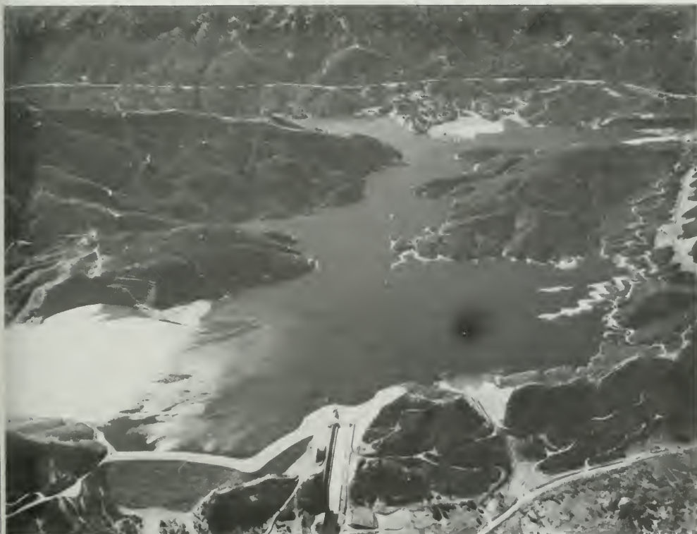
Figure 246. Aerial View—Cedar Springs Dam and Silverwood Lake
