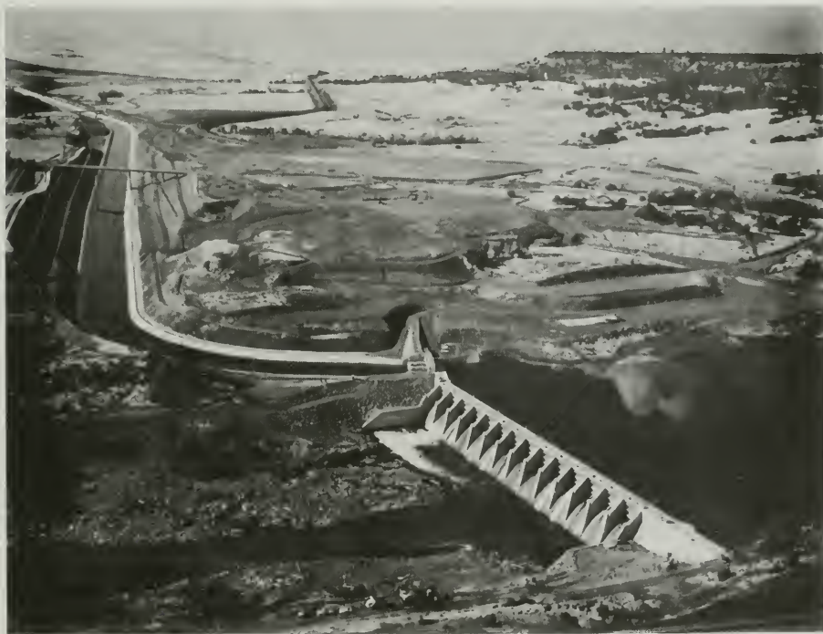
Figure 120. Aerial View—Thermalito Diversion Dam
