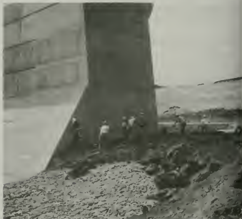
Figure 153. Hand Placement of Forebay Dam Adjacent to Powerplant Wingwall
