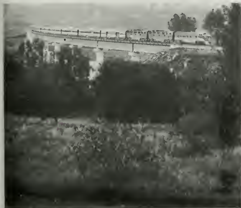
Figure 88. Feather River Bridge
