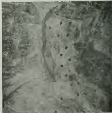
Figure 276. Rock Bolts in Dome of Outlet Works Gate Chamber
