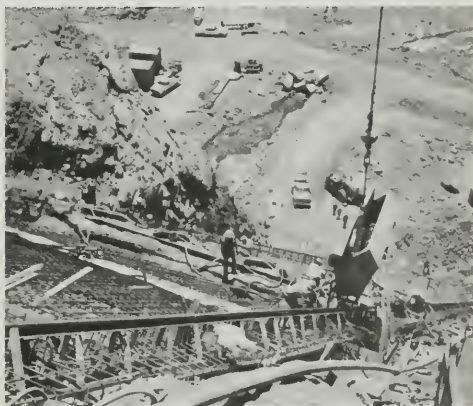
Figure 334. Concrete Placement in Spillway Chute Slab
