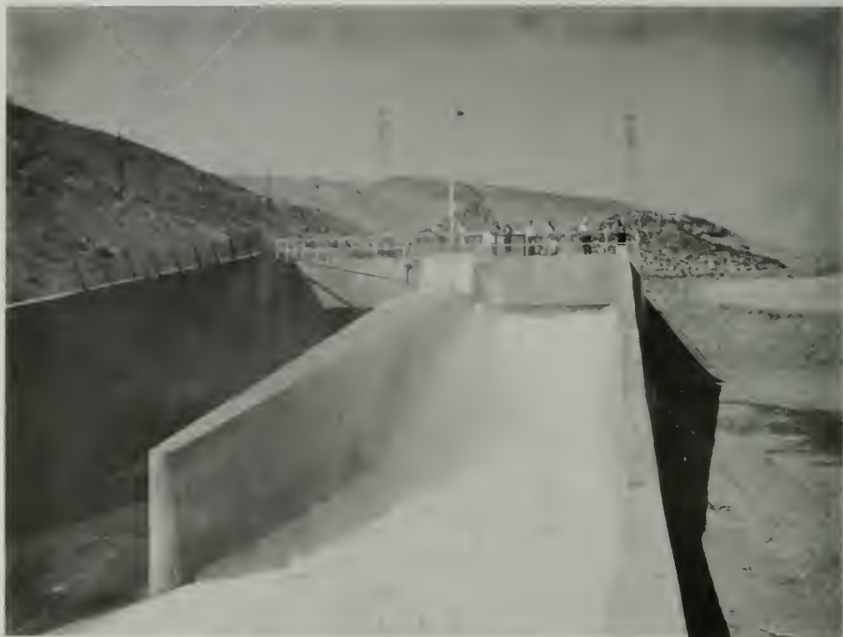
Figure 356. Outlet Works Stream Release
