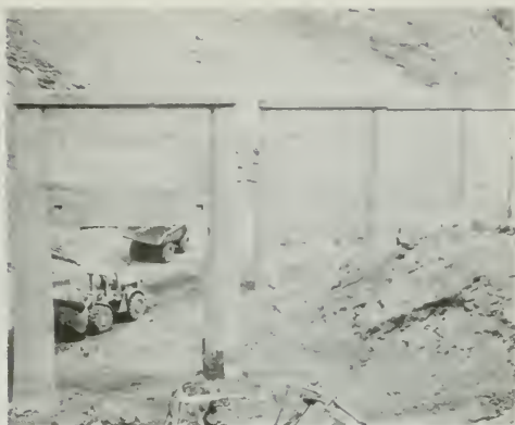
Figure 323. Old Highway 99 Bridge Bents Uncovered in Downstream Shell Area of Dam
