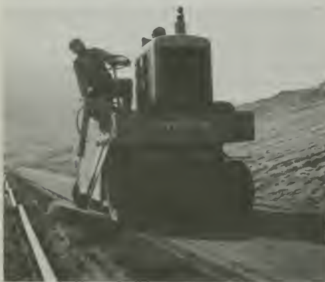
Figure 392. Compacting Soil-Cement
