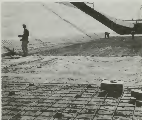
Figure 160. Reinforcing Steel Being Placed in Canal Invert
