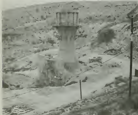
Figure 397. Low Intake Tower
