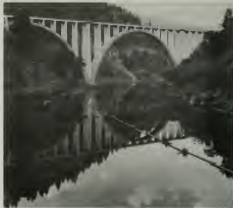
Figure 90. North Fork Bridge
