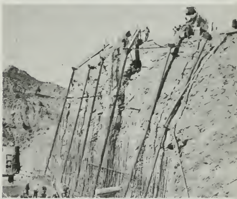
Figure 333. Concrete Placement in Spillway Headworks Invert
