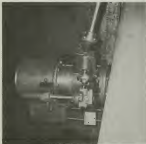
Figure 314. 8-Inch-Diameter Fixed-Cone Dispersion Valve
