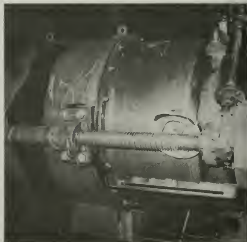
Figure 315. 36-Inch-Diameter Fixed-Cone Dispersion Valve
