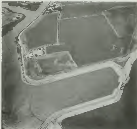
Figure 178. Control Structure and Inlet Channel Connection to West Canal and Old River (in background)
