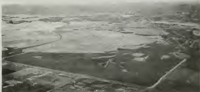
Figure 132. Aerial View—Thermalito Afterbay
