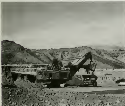
Figure 389. Loading of Pervious Borrow at Elizabeth Canyon
