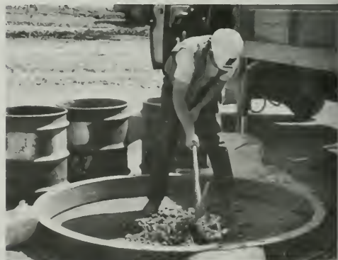
Figure 273. Performing Field Density Test on Zone 3 Material
