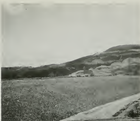
Figure 393. Downstream Cobble Slope Protection
