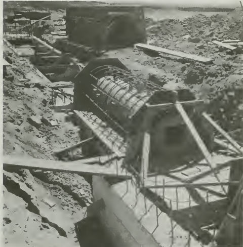
Figure 166. Pacific Gas and Electric Lateral Outlet Conduit
