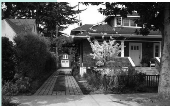
An old-fashioned driveway (a pilot project in the South Bay) allows more runoff to percolate (see sidebar).
