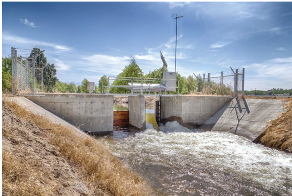
New Automated Check Structure in Packwood Creek
