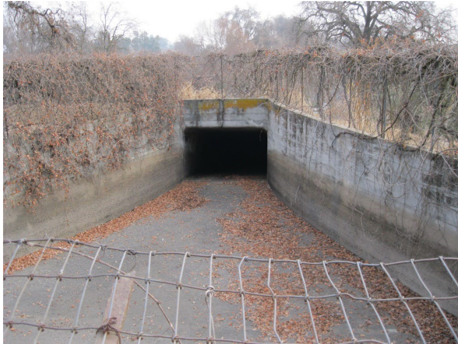
Inlet Structure – Lower Kaweah River Siphon
