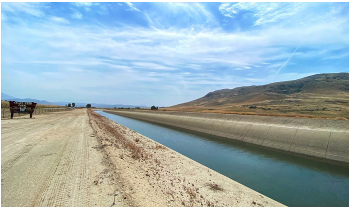
The Friant-Kern Canal near Fresno
