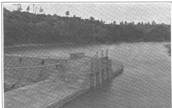
Dam and intake of canal on American River—Folsom power system.
