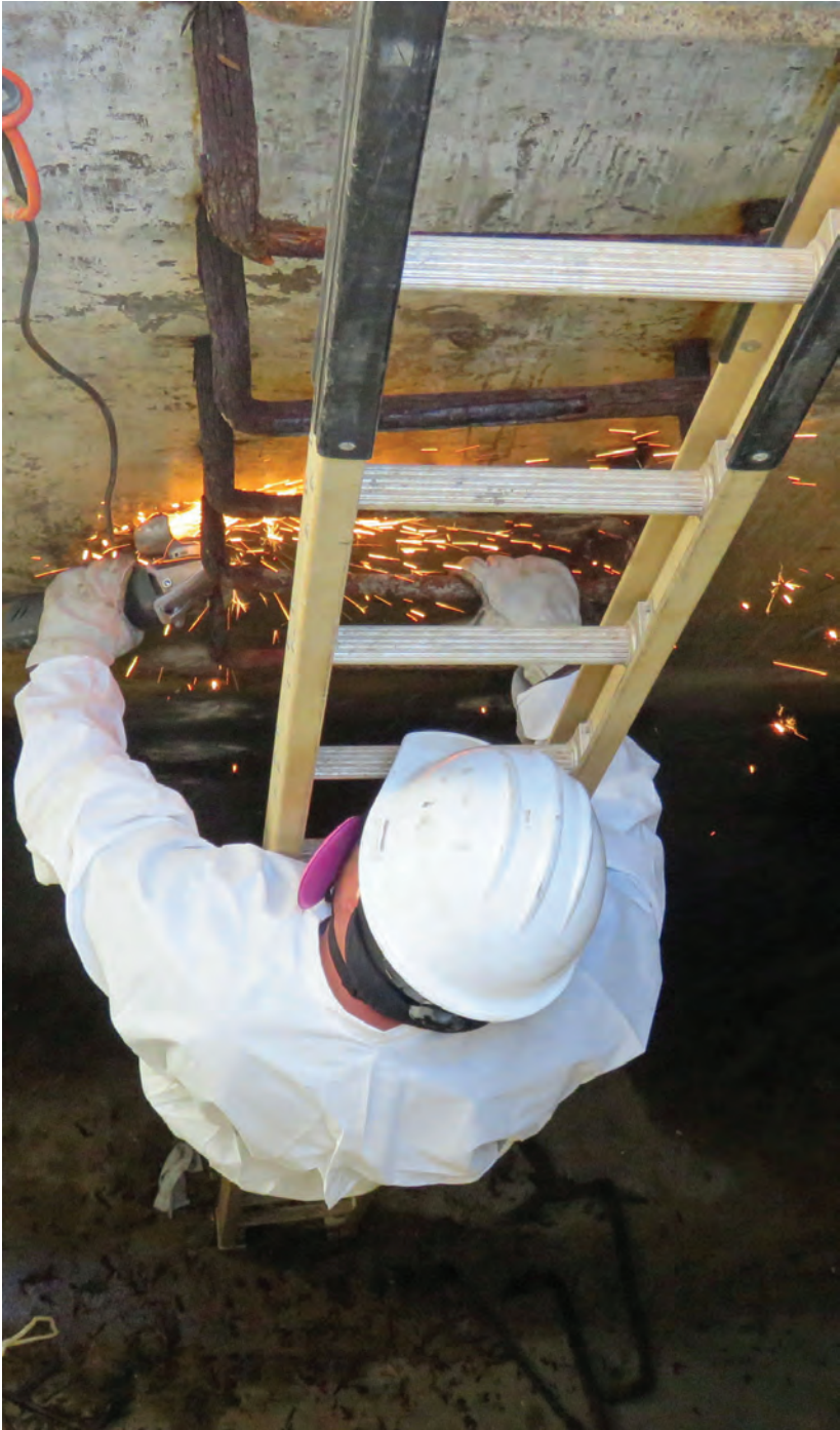
Removing deteriorated ladder rungs during a San Diego Pipeline shutdown.
