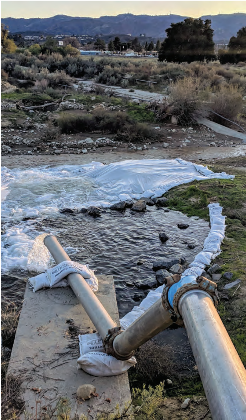
Dewatering the Foothill Feeder Pipeline into Placerita Creek during the January 2019 shutdown.
