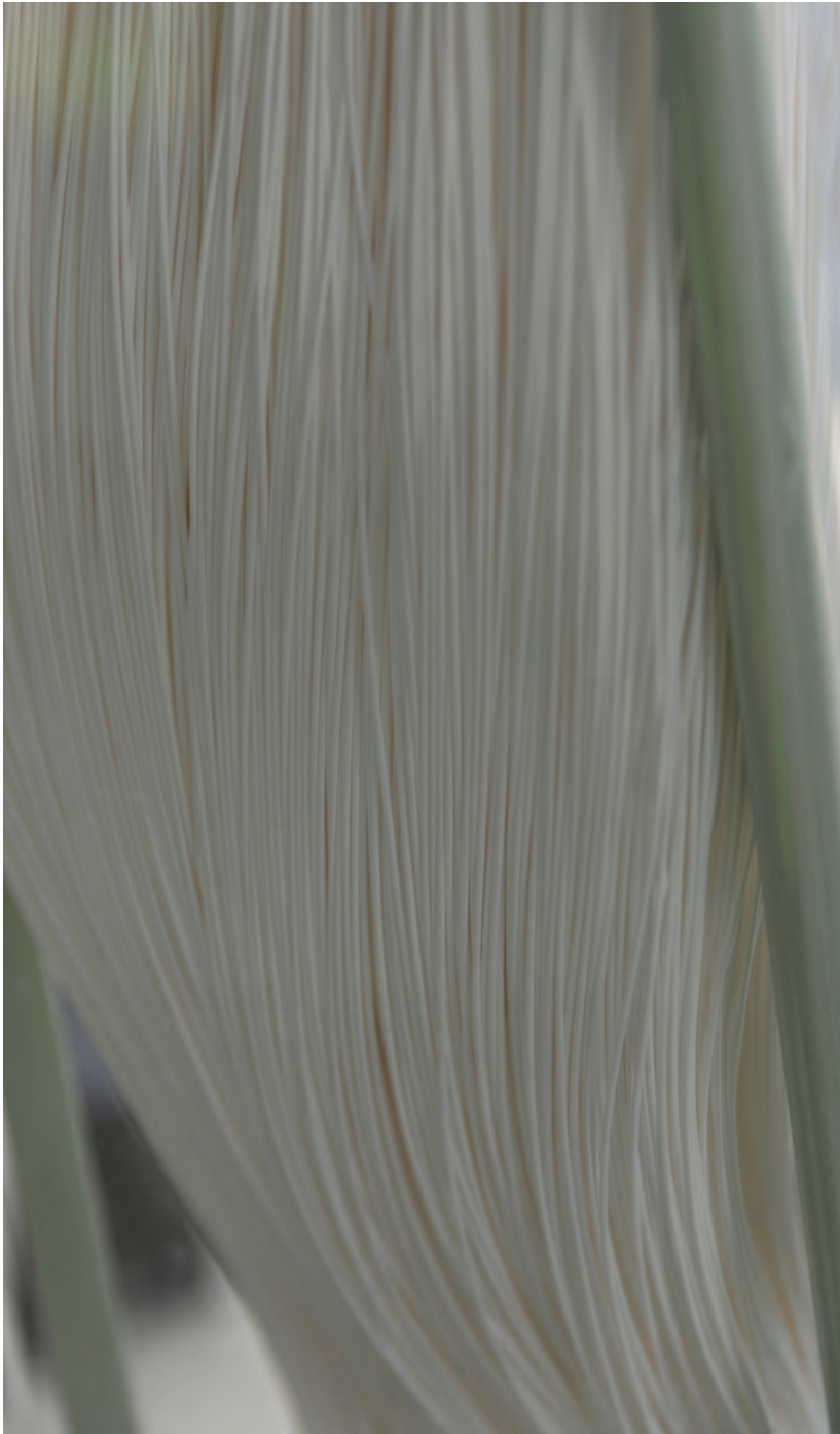
These straw-shaped membranes remove microorganisms at the Regional Recycled Water Advanced Purification Center, a 500,000-gallon per day demonstration facility in Carson finished in 2019.
