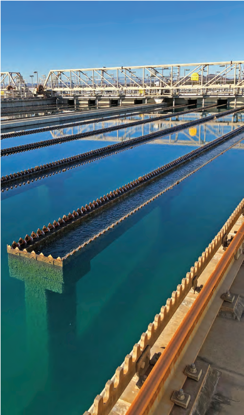
A settling basin at the Robert A. Skinner Water Treatment Plant in Winchester.
