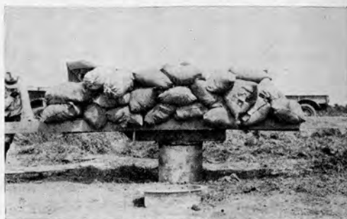
Pressing the inner tank into the soil.
