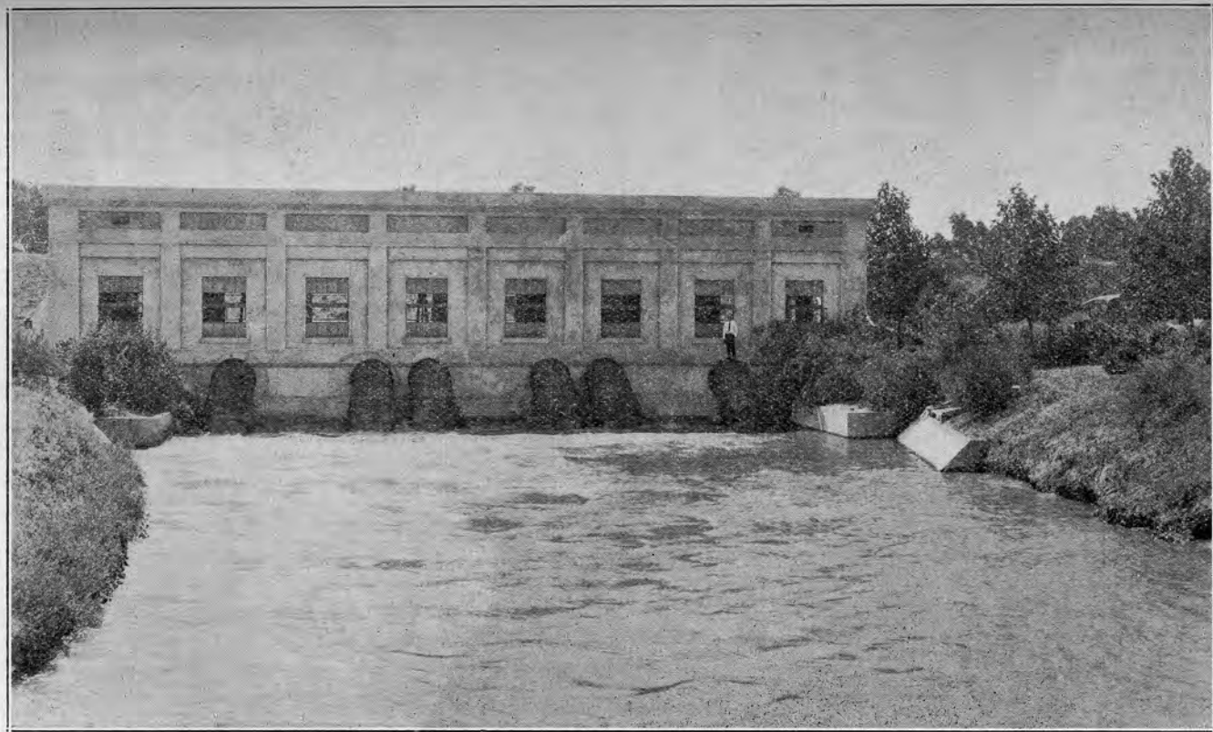
PLATE 3—One of the Largest Irrigation Pumping Plants on the Upper Sacramento River.
