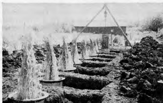
Excavation around inner tanks so that bottoms may be bolted on and the whole lifted inside the outer tanks.
