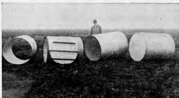
Inner and outer parts of asparagus tanks ready for installation.
