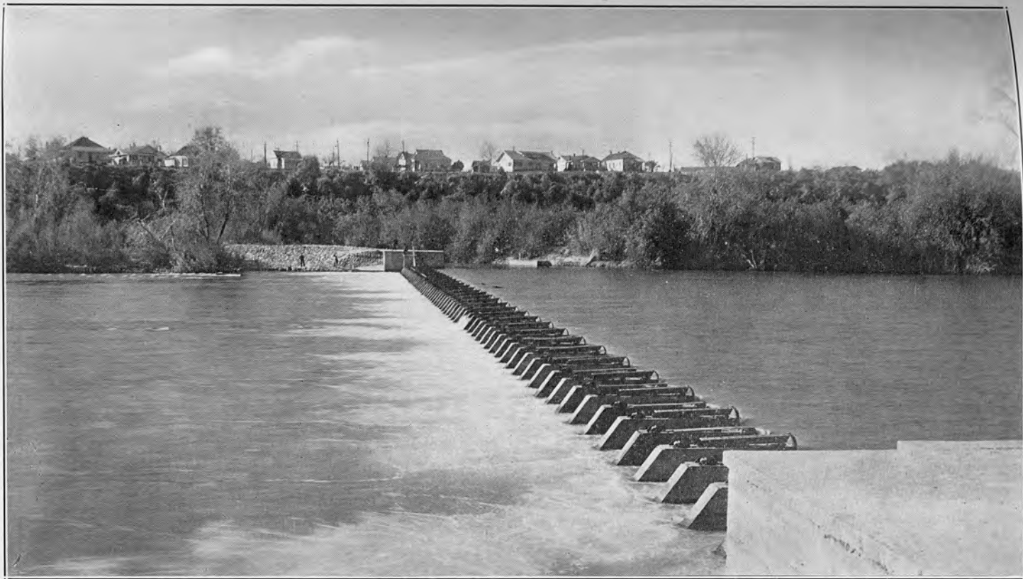
Collapsible weir across Sacramento River at Redding for diverting water into canal of Anderson-Cottonwood Irrigation District.
