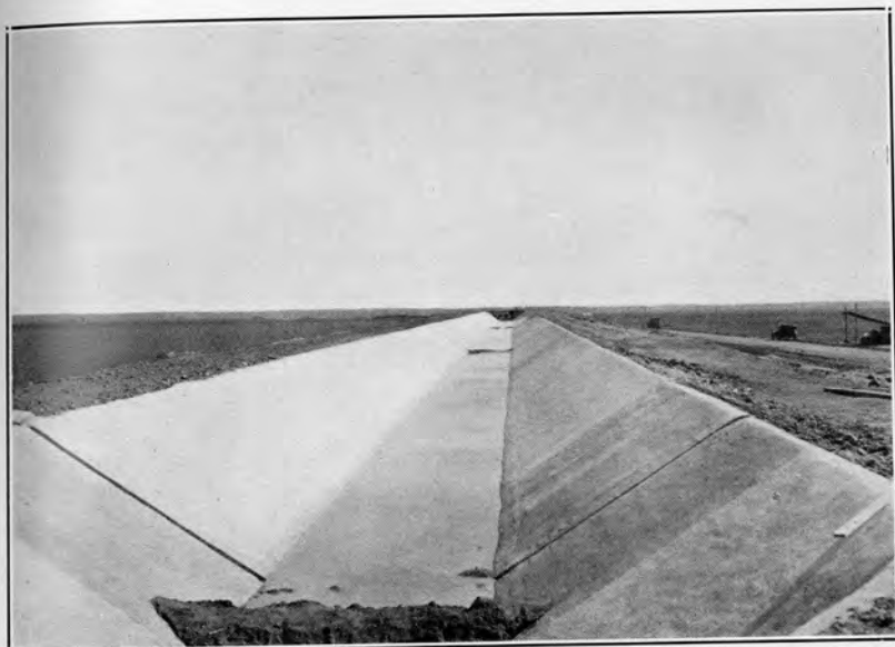
FIG. 2. Concrete-lined main canal, West Stanislaus Irrigation District.
