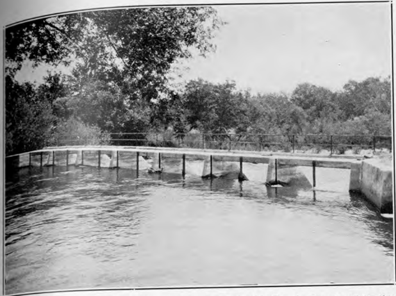
FIG. 1. Weir across Kings River at head of Gould Canal, Fresno Irrigation District.
