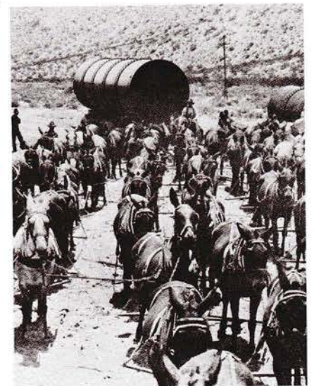
36-ton sections of the Los Angeles Owens River Aqueduct were hauled into position by mule teams
