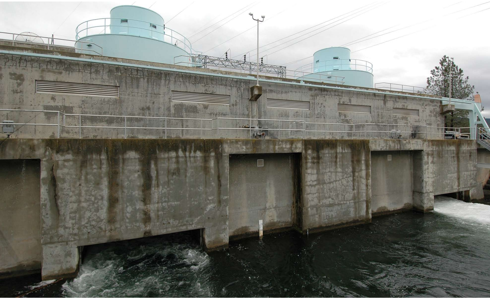
The Tuolumne River generates hydropower at Moccasin Powerhouse.
