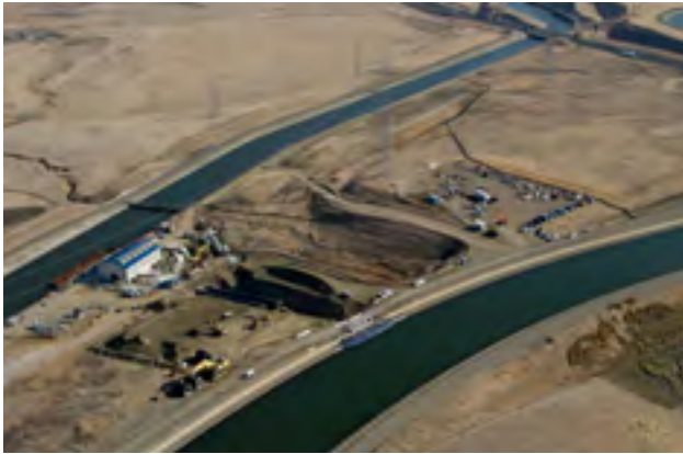
A $29 million intertie was completed in 2012 to link the SWP's California Aqueduct and the CVP's Delta-Mendota Canal, to enable increased flexibility in the projects' operations.
