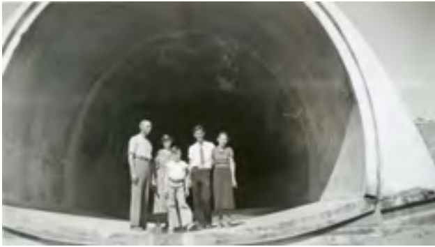
Construction of MWD's Colorado River Aqueduct in the 1930s, tunneling through the San Jacinto Mountains. Photo courtesy of Banning Library District.
