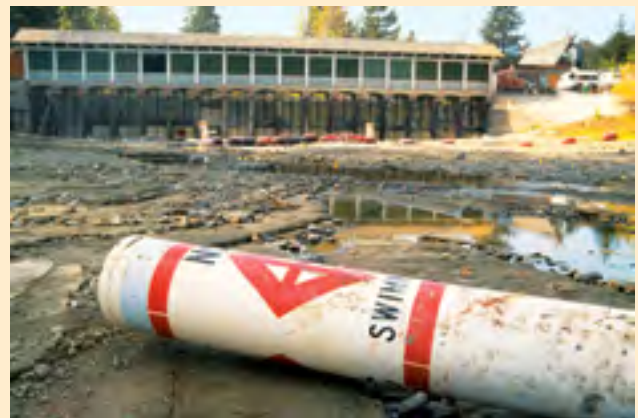
Lake Tahoe periodically falls below its natural rim during drought conditions, leaving USBR's dam on the lake's outlet to the Truckee River high and dry.
