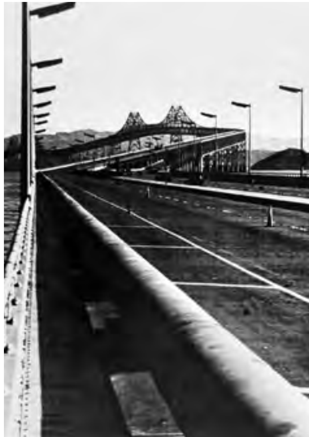
An iconic image from the 1976-77 drought was the temporary emergency pipeline constructed across the San Rafael Bridge to bring imported water into southern Marin County.
