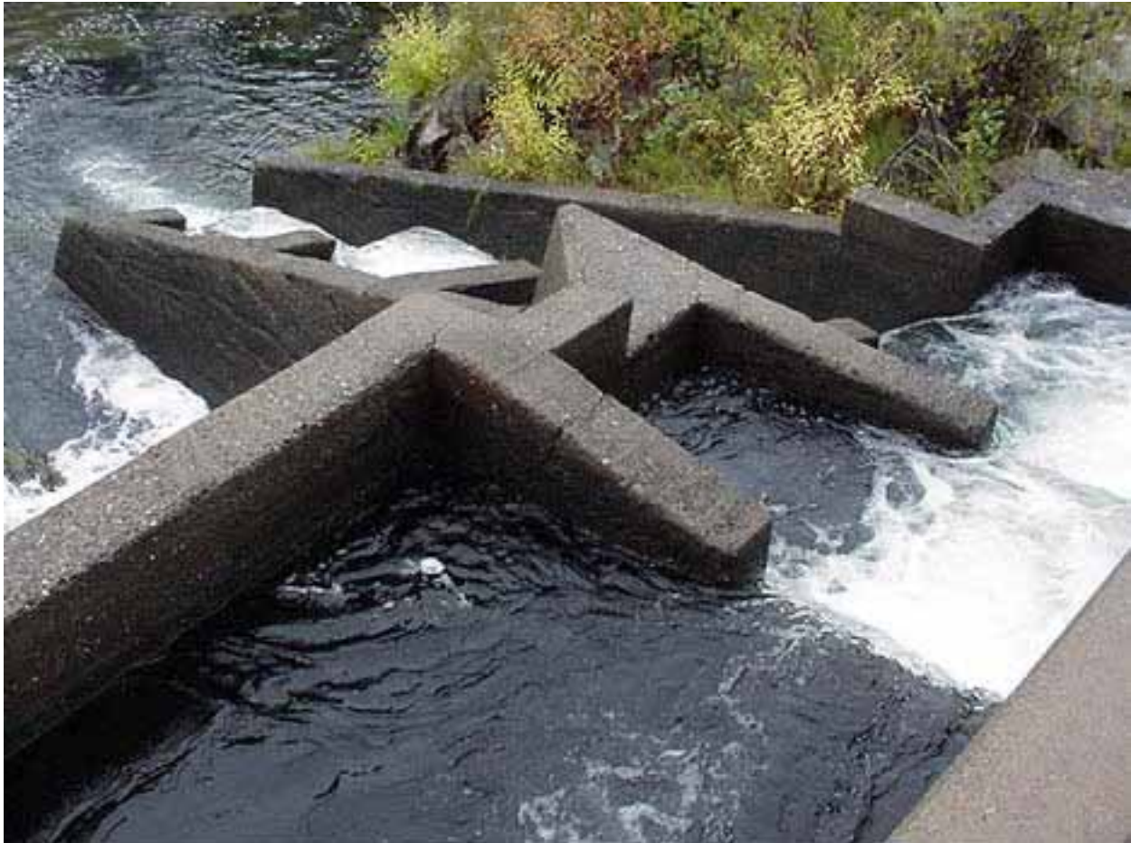
Photo 4-15 Cosumnes River—fish ladder at North Granlees Dam (Retrofit in 2003)
