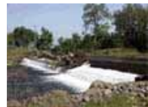
Photo 4-9 Deer Creek—Stanford-Vina Ranch Diversion Dam /Photo
