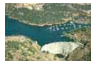
Photo 4-12 Yuba River–Harry L. Englebright Dam / CALFED photo
