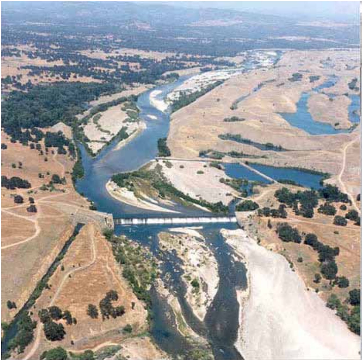
Photo 4-11 Yuba River—Daguerre Point Dam
