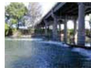
Photo 4-27 Tuolumne River—Dennett Dam (Stanislaus County)/DWR Photo
