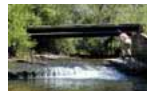
Photo 4-17 Dry Creek— pipeline on Secret Ravine (Sacramento and Placer counties)/DWR photo
