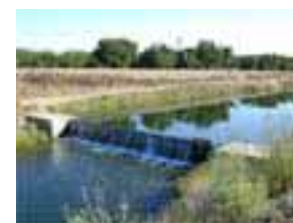
Photo 4-22 Mormon Slough—flashboard dam /DWR photo
