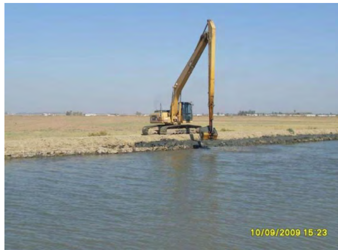
Figure 4-19. Desilting the Outside Canal and raising embankments remediated subsidence downstream from Russell Avenue (photograph courtesy of Chris White, Central California Irrigation District).
