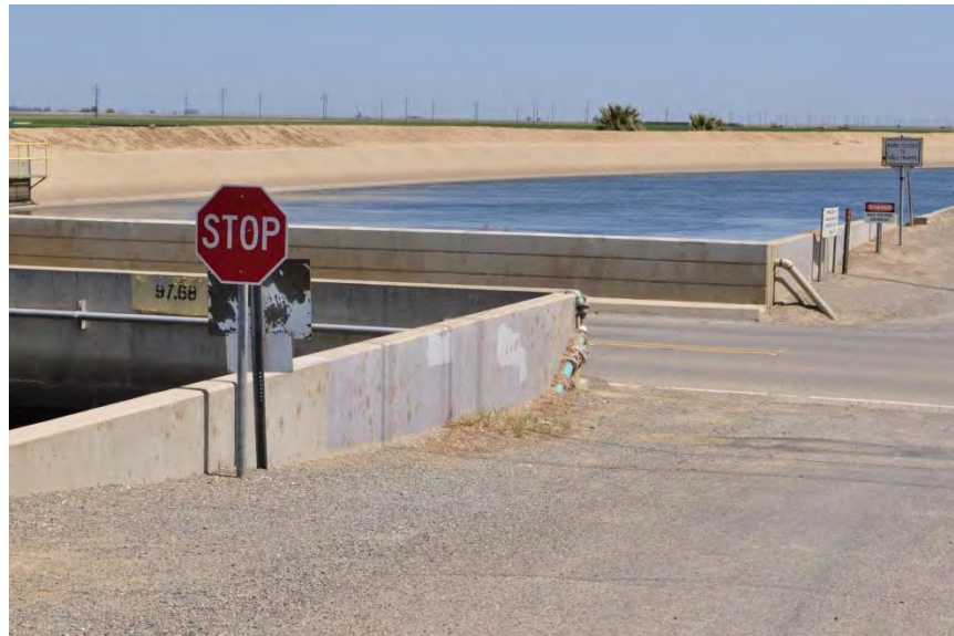
Figure 4-15. Delta Mendota Canal at Russell Road bridge north from Mendota, CA, looking downstream. Raised wing walls prevent water from overtopping Russell Avenue.
