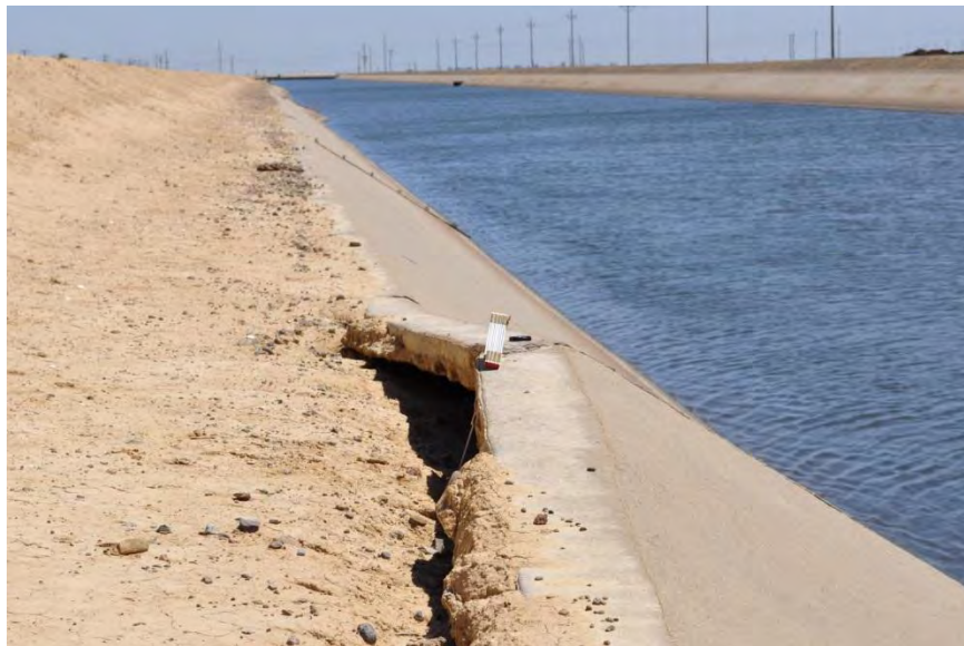
Figure 4-18. Ruptured lining of the Delta Mendota Canal in the subsiding area about 0.6 miles upstream from the Russell Avenue bridge.
