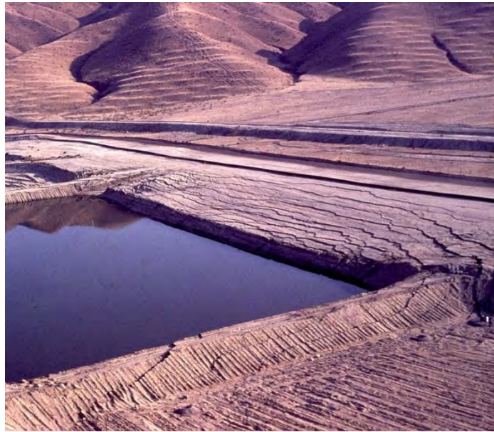
Figure A-7. Flooding basin in Kern County, California, used to “presubside” sediments subject to hydrocompaction along the proposed route of the California Aqueduct. Note the step-wise, differential subsidence between tension-fissured scarps on the basin dikes. To prevent deleterious effects of hydrocompaction, large sections of the alignment of the Aqueduct were precompacted in this manner prior to construction (photograph by Joseph F. Poland, October 13, 1965).
