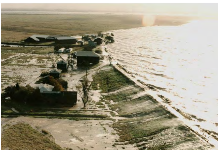
Figure A-5. Wind-whipped waves spilling over the levees on the north side of Jersey Island in the Sacramento-San Joaquin Delta December 3, 1983 (photo by Kenneth L. Kjeldsen).
