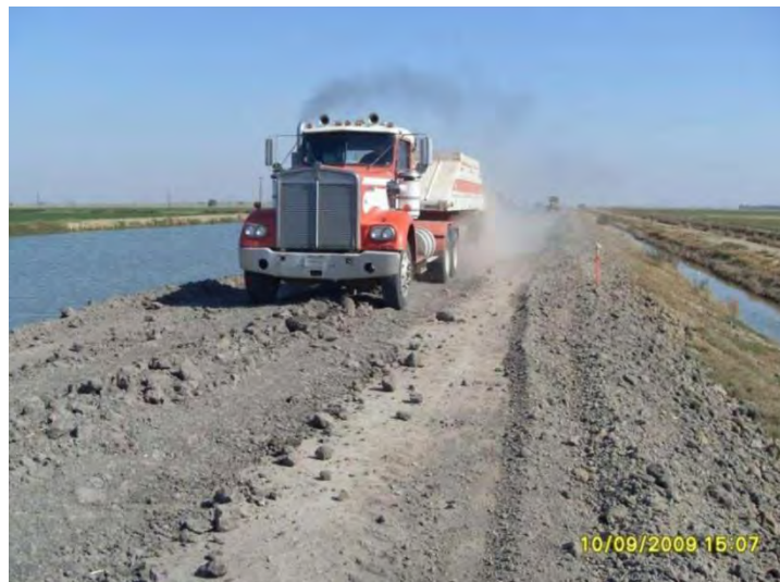
Figure 4-20. Importing fill material to raise embankments in subsided areas of the Outside Canal (photograph courtesy of Chris White, Central California Irrigation District).
