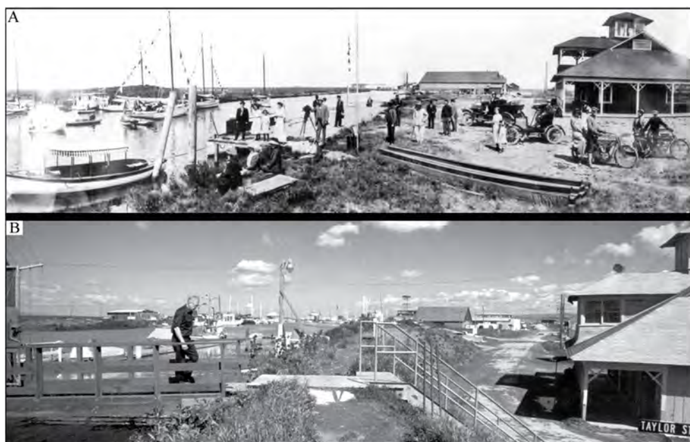
Figure 4-4. The South Bay Yacht Club at Alviso, California in A) 1914, before dikes were necessary to prevent flooding and B) 1978 after dikes were constructed to prevent bay water from flooding areas near the yacht club that had subsided to 10 feet below sea level. The yacht club headquarters stands on the right side of each photograph (photographs courtesy of Santa Clara Valley Water District).
