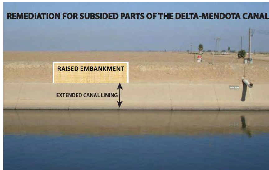
Figure 4-17. Raised canal linings and embankments upstream from Russell Avenue remediated the water-ponding effect of land subsidence.
