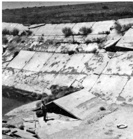
Figure A-8. Hydrocompaction damage to a canal test section in the west-central San Joaquin Valley. The earthfill embankment cracked and settled, the concrete lining and earthfill embankment separated, and the 4-in thick concrete lining cracked and buckled after the test section was flooded. (Photograph from Prokopovich, 1983). Precompacting the alignment of the California Aqueduct by flooding helped to prevent similar damage.
